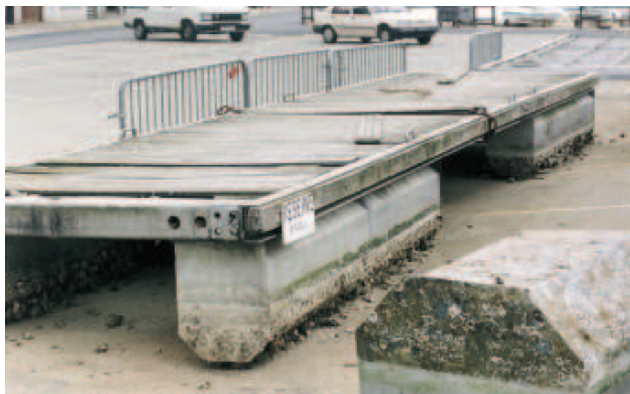
MARINA PONTOON AND FLOATS MADE OF 5754
