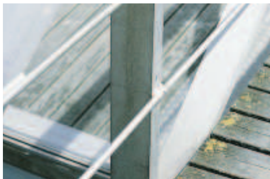
WELDMENT ON A GANGWAY
