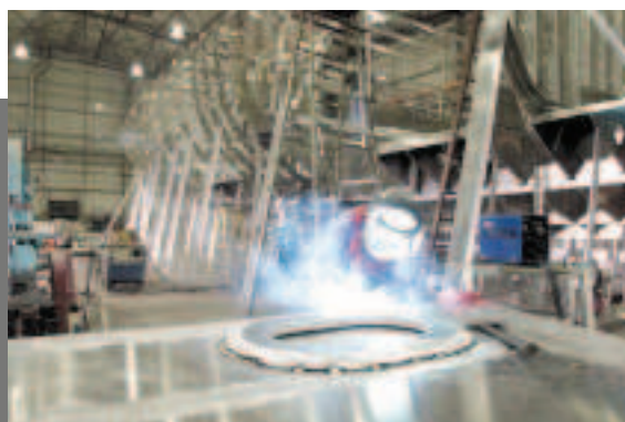
WELDING A HATCHWAY FRAME
