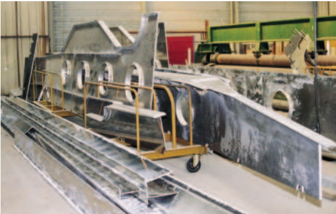
HIGH INERTIA BEAM FABRICATED BY WELDING SHEETS
